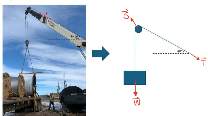
2) (20 points) Assume the acceleration due to gravity is  $g = 9.8 \text{ m/s}^2$ . Determine the weight of the 500 kg load.
